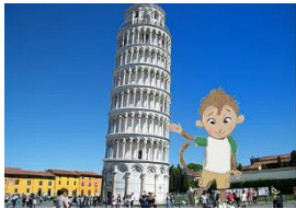
Leaning Tower of Pisa
